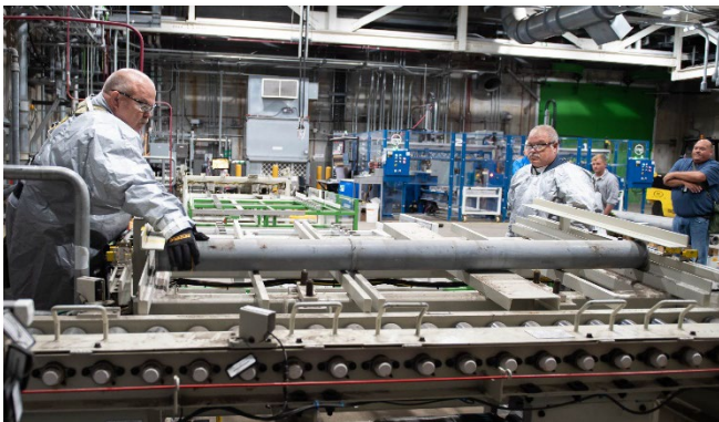
Blue Grass operators place the first M55 rocket containing GB nerve agent on a conveyor to begin the destruction process.
